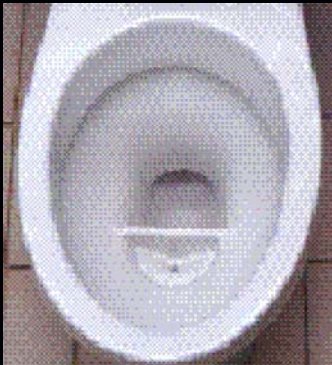
Urine diversion toilet with dual flush function
