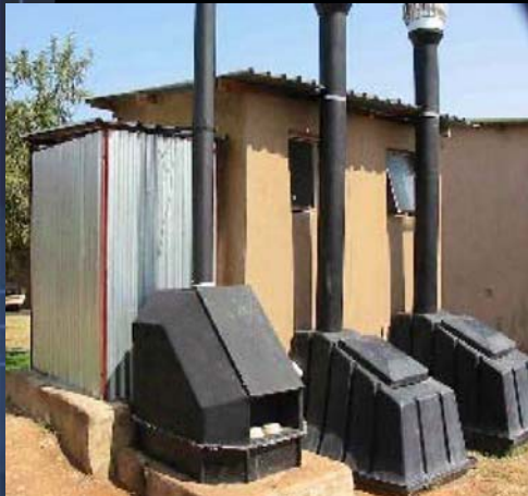
Without urine diversion; Solid and liquid is separated at the initial stage of entering
