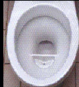
Urine diversion toilet with dual flush function
